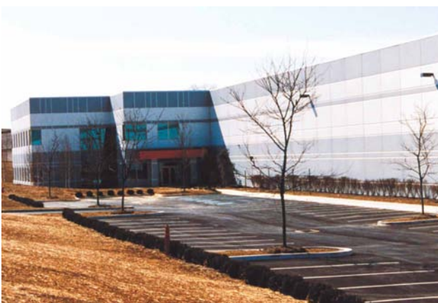
Figure 1.2.11 Precast and prestressed concrete flat panels are used for warehouse walls. Hollow-core slabs may also be used in this application.
