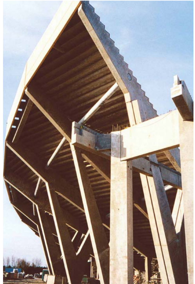
Figure 1.2.38 Special framing is handled easily with precast concrete, eliminating expensive field formwork.
