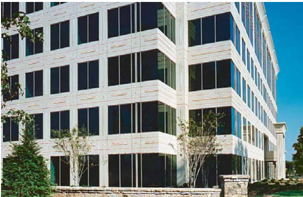
Figure 1.2.34 Spandrel panels spanning from column to column can be load-bearing or solely architectural.
