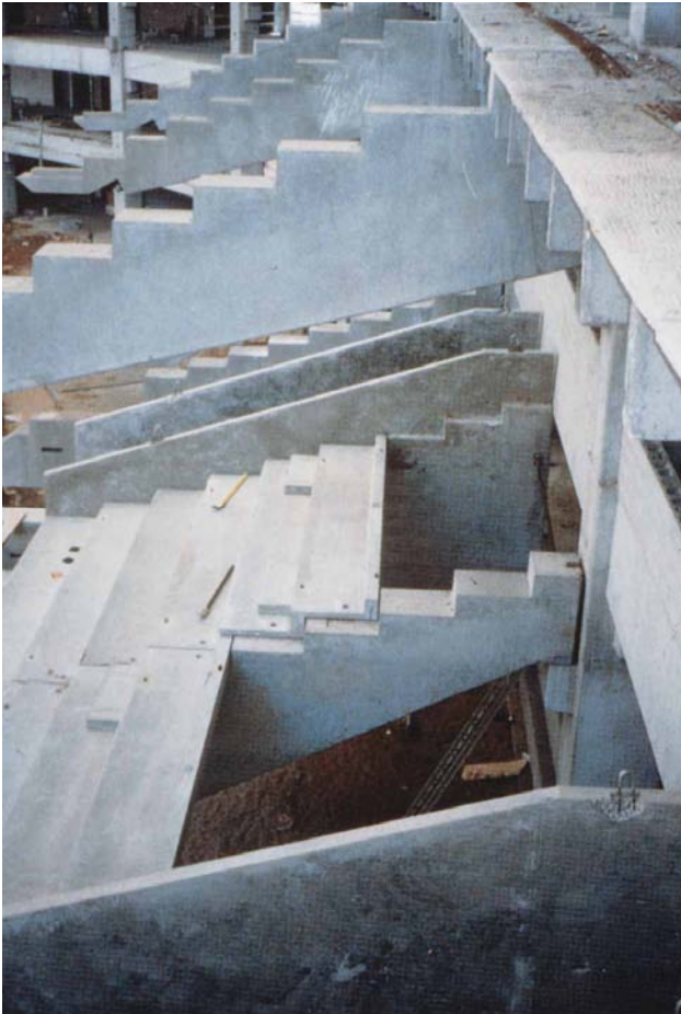
Figure 1.2.36 Precast concrete risers, raker beams, columns and mezzanine floors play a prominent role in stadium construction.
