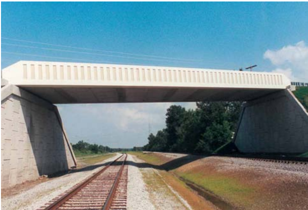
Figure 1.2.45 The use of large, hollow edge beams with solid floor slabs and field post-tensioning provided a 110-ft span with only a 14-in. structure depth in this through-girder solution.
