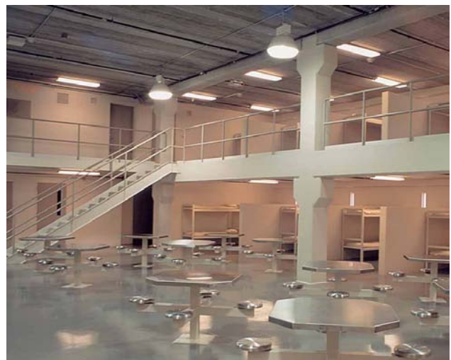
Figure 1.2.29 Interior finishes of prisons are durable and maintenance free. Soundproof and fire resistant, precast concrete adds to security and limits vandalism.
