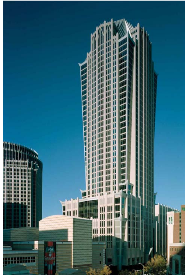
Figure 1.2.31 Architectural precast concrete provides a striking facade for the landmark Hearst Tower in Charlotte, North Carolina.
