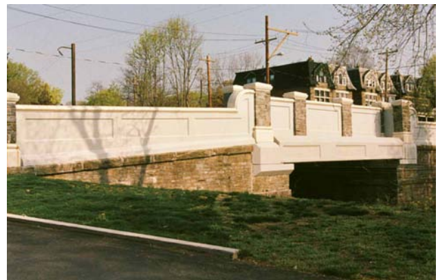
Figure 1.2.48 A short span bridge over an electrified railroad blends well with a historic residential area. The bridge sits on original stone abutments nearly 200 years old.
