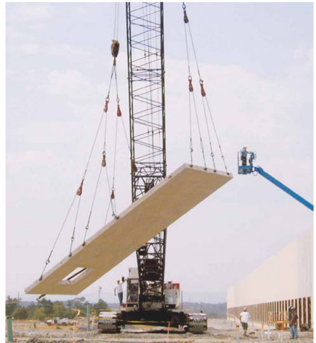
Figure 1.2.13 Precast concrete insulated sandwich wall panels provide excellent insulation for cold storage facilities. Smooth interior finishes make these panels an excellent choice for food processing plants.
