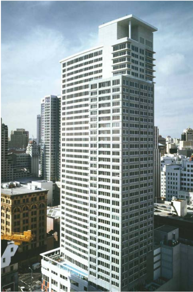
Figure 1.2.30 The Paramount building in San Francisco is 39 stories tall. It is the tallest precast, prestressed concrete framed building in a high seismic region.
