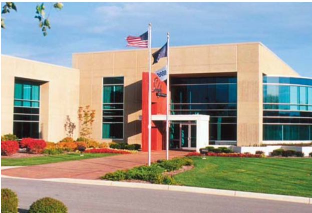
Figure 1.2.10 The light industrial office structure is erected and put into service quickly using insulated precast concrete sandwich panels.
