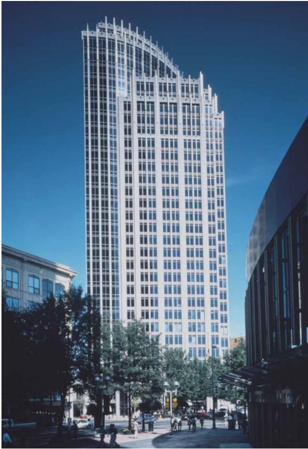
Figure 1.2.33 Repetition of size and shape, which allows multiple form use, is a key to economy.
