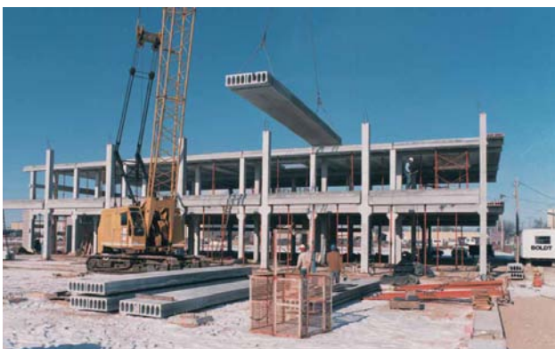
Figure 1.1.3 Erection of hollow-core deck members.
