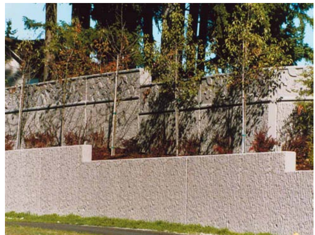
Figure 1.2.47 Precast concrete soundwall provides aesthetics and protects residential neighborhood from highway noise.
