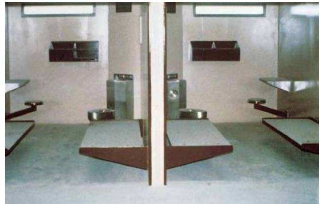
Figure 1.2.28 Box module cells are often supplied with electric conduit and boxes, furniture, window and door embedments, and mechanical and plumbing chases cast in.
