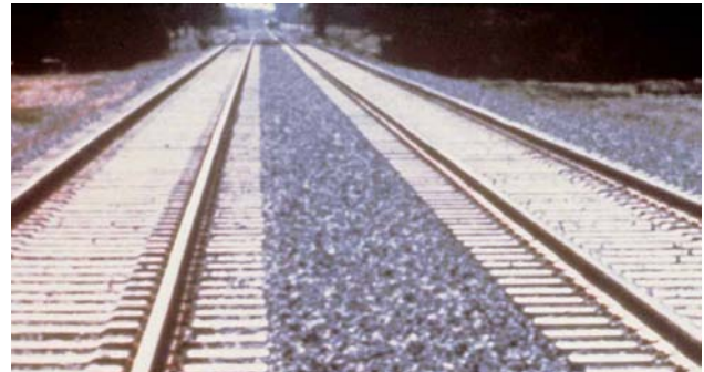
Figure 1.2.52 Precast and prestressed concrete has proven to be a viable alternative to timber for railroad ties.
