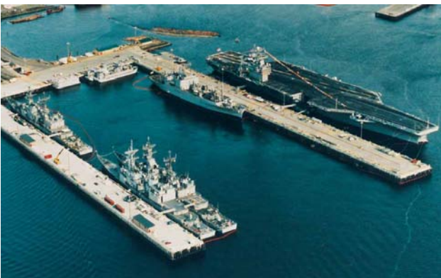
Figure 1.2.50 This breakwater/pier structure for the United States Navy incorporates piles, deck panels, utilidor lids, and vertical panel elements. Economic analysis shows precast and prestressed concrete to be the best solution.
