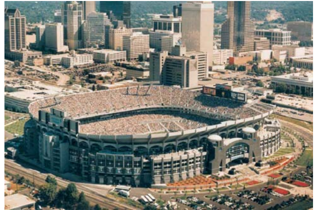
Figure 1.2.35 This major sports stadium was built using total precast concrete after evaluating other systems.
