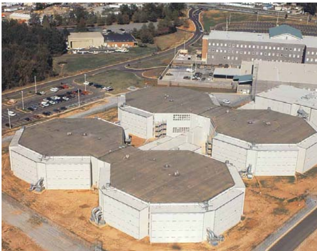
Figure 1.2.26 The repetitive nature of cell layout and the typical quick occupancy requirements make precast concrete an ideal solution to prison overcrowding.
