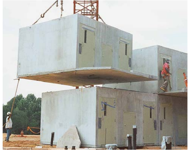
Figure 1.2.27 Precast double-cell module being lifted into place.
