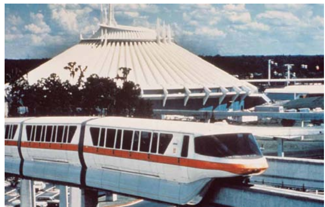
Figure 1.2.53 Famous amusement park building in background has precast and prestressed roof and walls. Monorail guideway is also precast and prestressed concrete.
