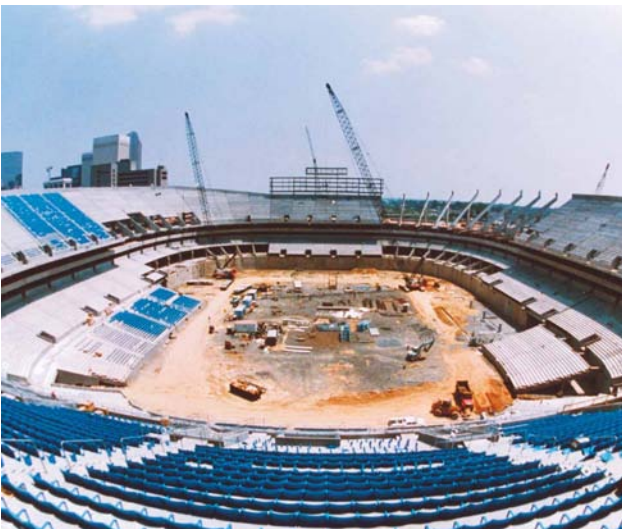
Figure 1.2.37 Fast track construction allows compressed schedules. Site preparation and component manufacturing can take place simultaneously. Multiple erection crews speed erection.
