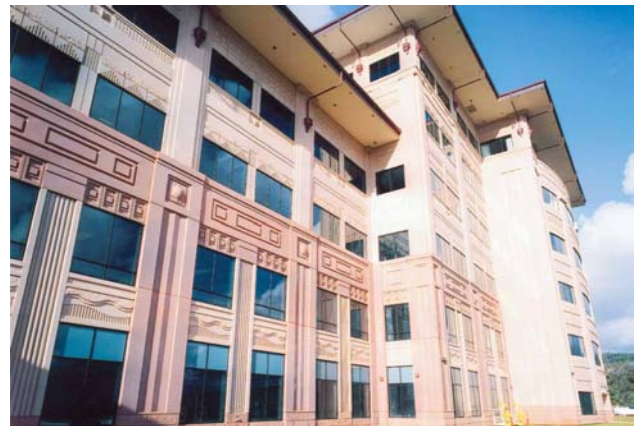
Figure 1.2.32 The moldability of architectural precast concrete allows for an infinite number of sizes and shapes.
