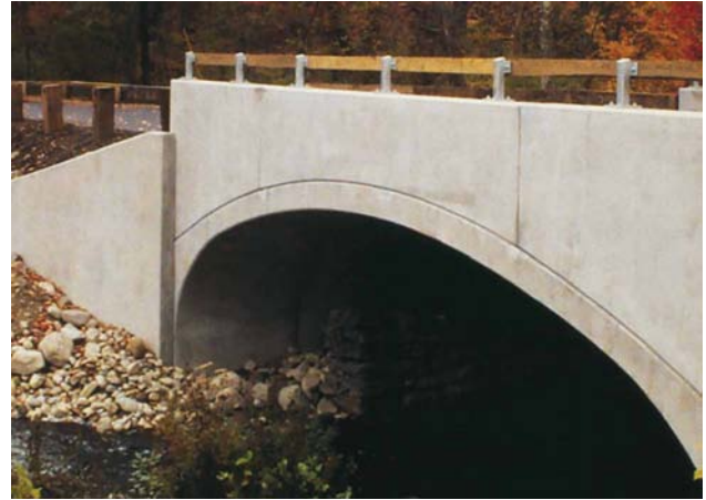
Figure 1.2.46 Precasting this arched culvert and its footings and wing walls allowed quick erection with little site disruption and no field formwork.
